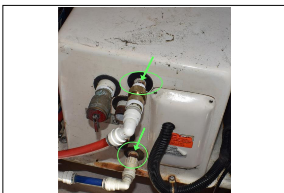
Corroded Fittings
