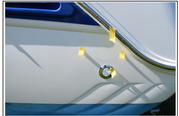
Gel Coat Repair Area
