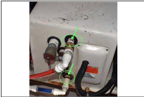
Corroded Fittings
