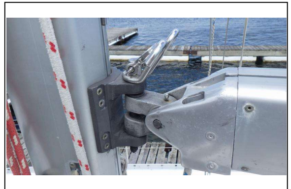
Improper Sized Pin
